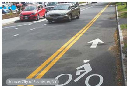
contraflow bike lane
