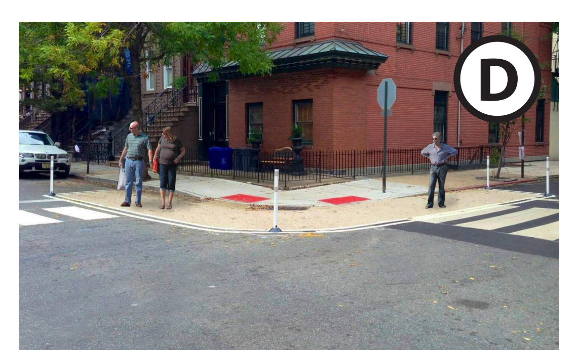
Curb Extensions visually narrow the street, reduce the crossing distance for pedestrians and bicyclists, and can increase the amount of space for street furniture and trees. Credit: RBA
