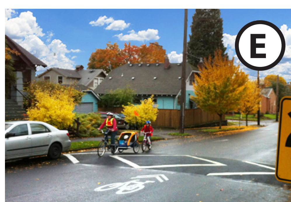
Speed humps prevent motor vehicles from speeding through neighborhoods and generally have a negligible impact on the amount of time it takes for residents to access their property. Credit: NACTO
