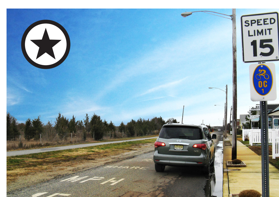
Ocean City, NJ has set a 15 mph speed limit on the Haven Avenue Bicycle Boulevard to reduce the speed differential between motor vehicles and bicycles. Credit: RBA
