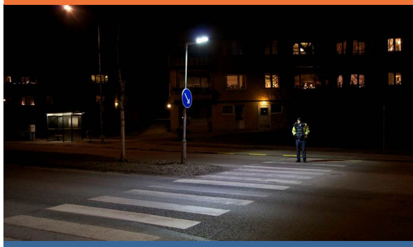
At this mid-block crossing, the pedestrian is illuminated for oncoming vehicles. (Credit: LowerEnergyDesigns.com)
