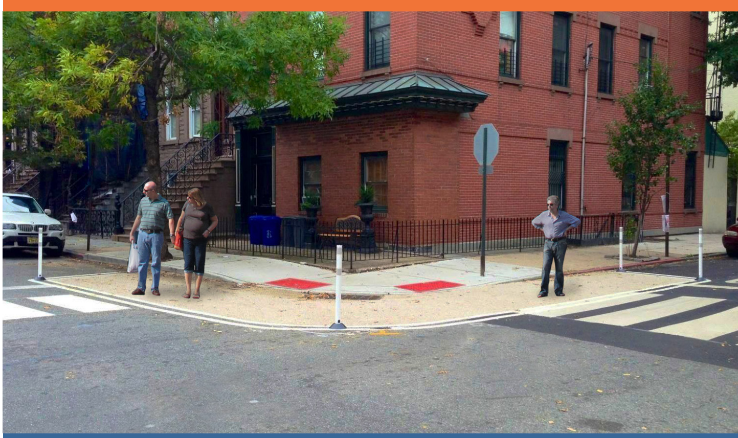
A painted (epoxy) curb extension with pylons was an effective interim or low-cost solution in Hoboken, NJ.
