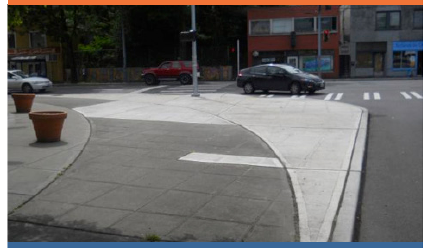
This modified curb radius reduces the speed of turning vehicles and shortens the pedestrian crossing. (Credit: Michael Hintze)
