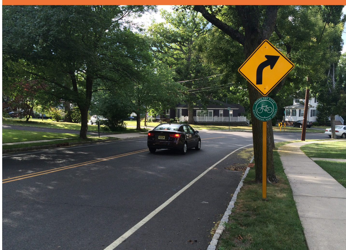
Adding shoulder striping to this street narrowed the travel lanes and provided space for bicyclists.
