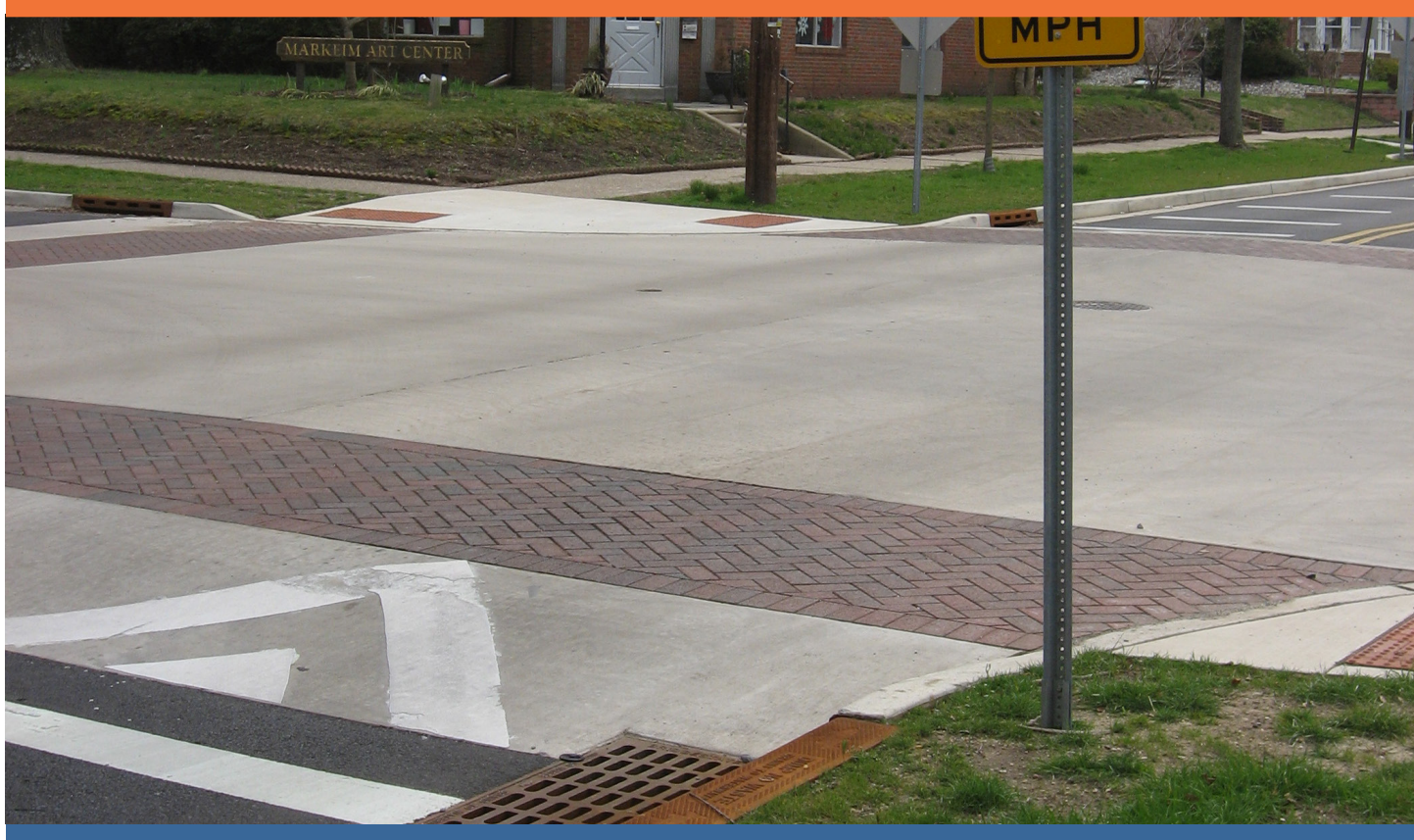
A raised intersection in Haddonfield, NJ. (Credit: VTC)
