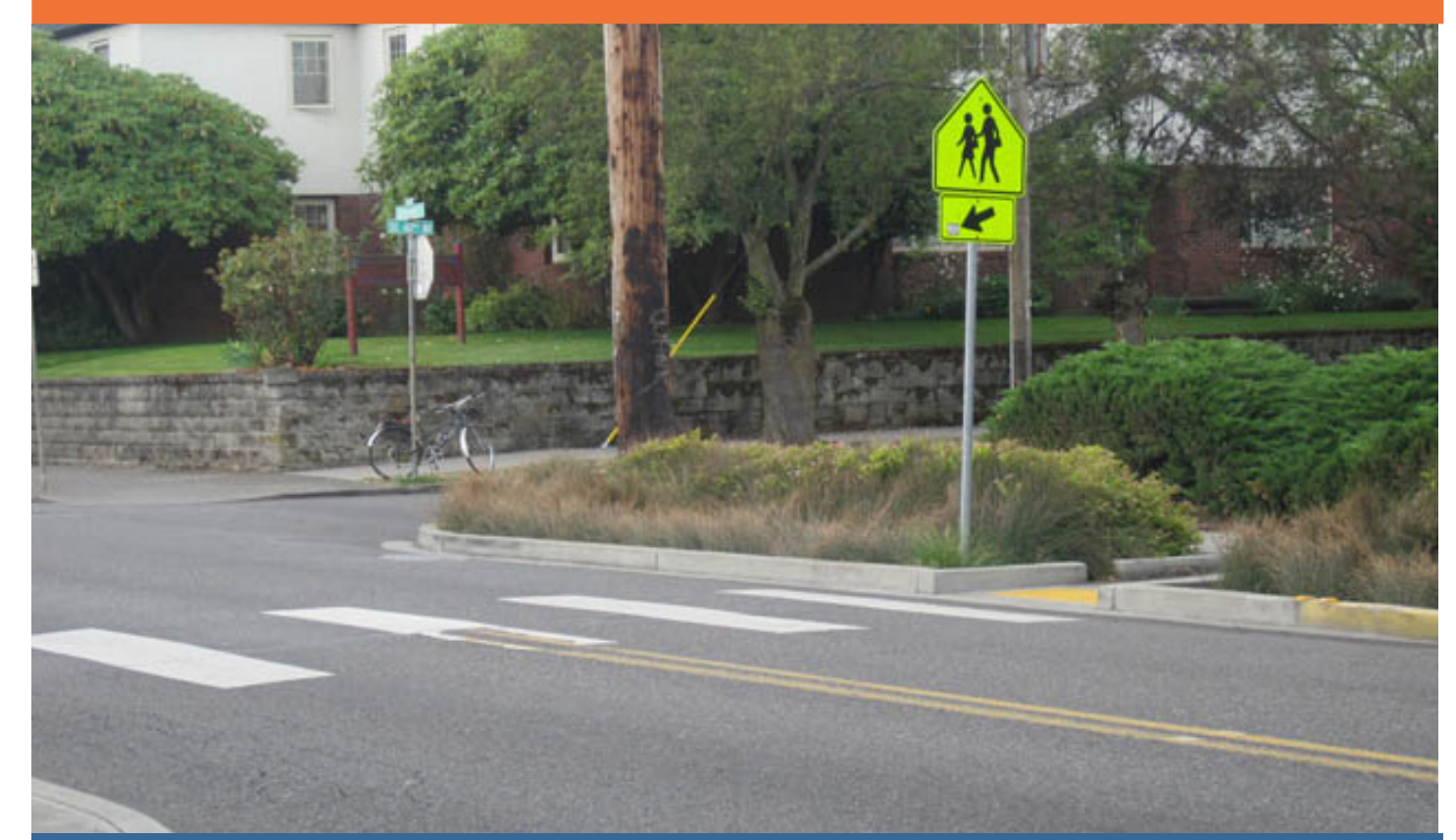
This curb extension assists pedestrians in crossing the street while filtering stormwater runoff. (Credit: NACTO)
